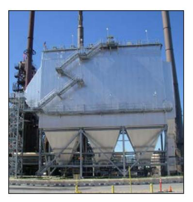
Emissions from the stack are guaranteed not to cause a discharge into the atmosphere of any gases that exhibit greater than 5% opacity when any four (4) of the twelve (12) electrical sections are out of service.
