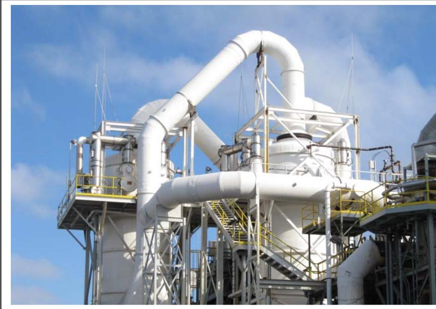
**Figure 5: Two-Stage Membrane WESP Modules at Climax Acid Plant**
