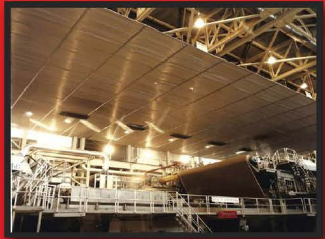
PAPER MACHINE ROOM FALSE CEILING
